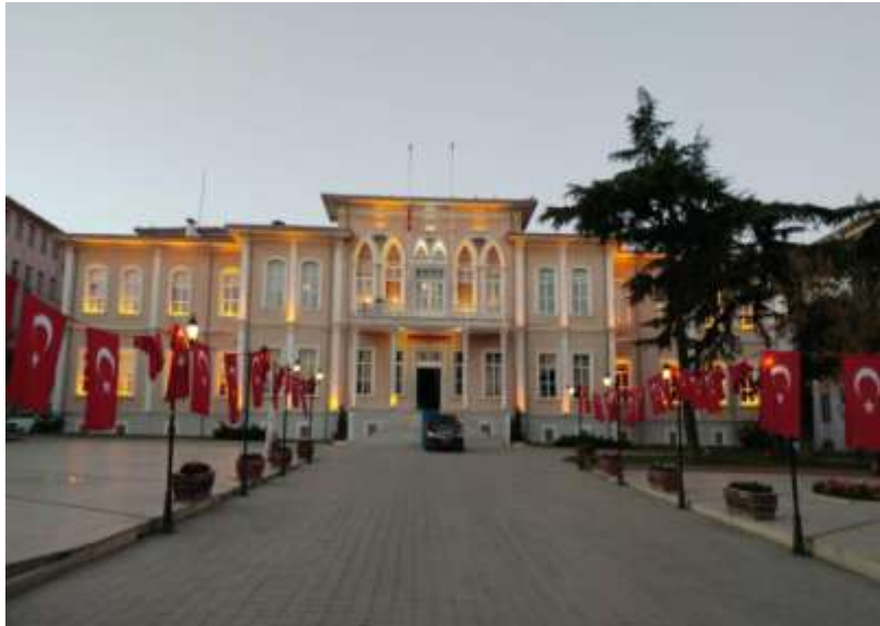
Figure 1. Government Building (Photos by Sermin Sentürk, 2016)
