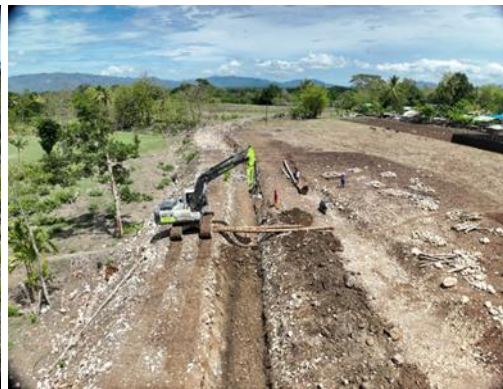
Figure 4.2 Irrigation Channel Excavation Work
