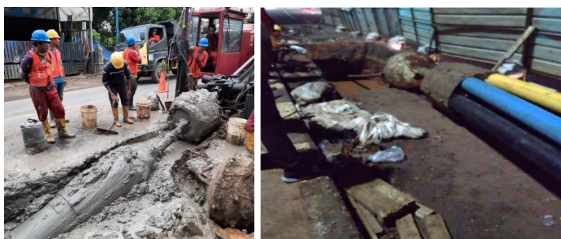
Figure 1: HDD Method PE Installation for Water Supply System and Medium/High Voltage Cable Lines
