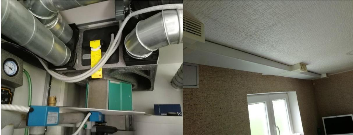
Figure 8: View of the recuperation ventilation unit and air ductwork in the measuring room
