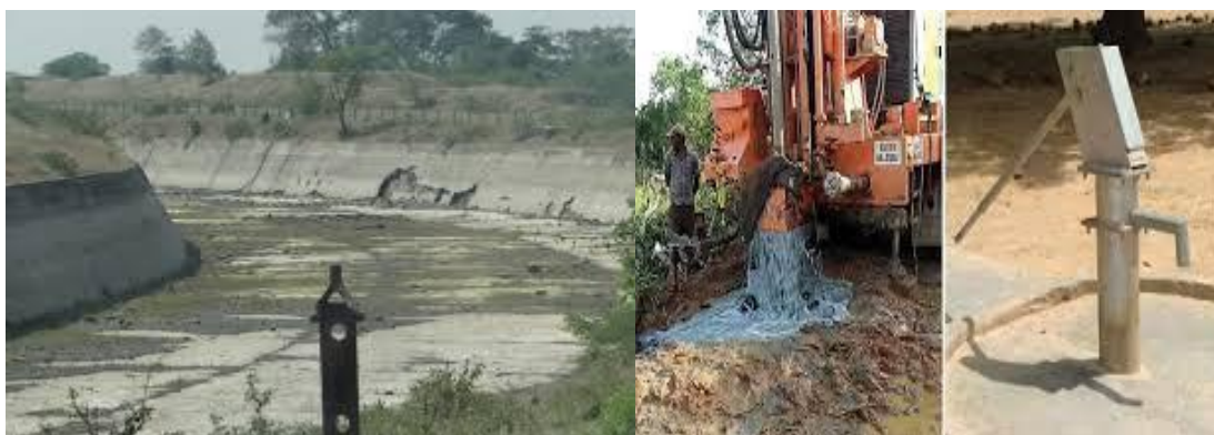
Diagram 1: canal under construction (left) & usage of borewell and handpump (right)
