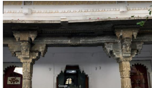
Figure 16: Timber Beams, Bagore ki Haveli (Source:
