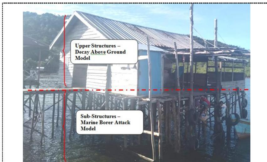
**Figure2:** Building structure decay modeling
