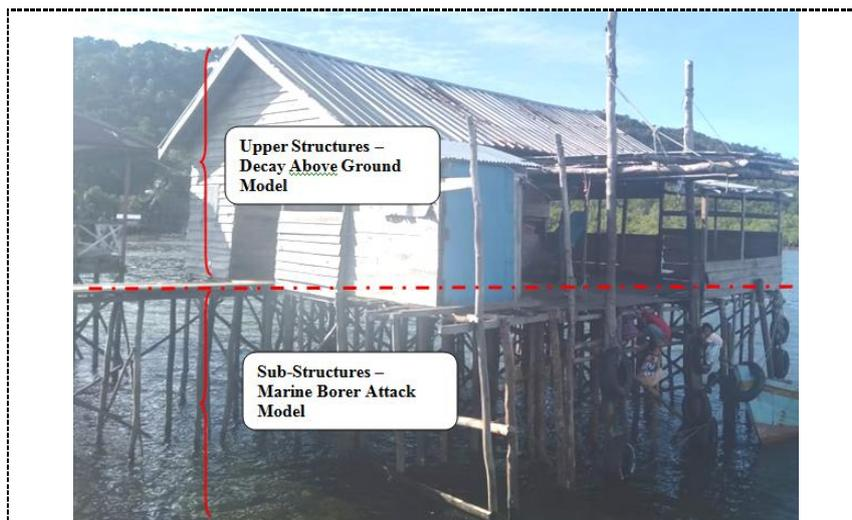
**Figure2:** Building structure decay modeling
