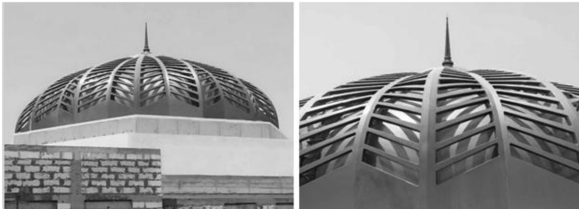
Fig. 7. Convention center GRP Dome, Location: Bahrain, Client: Confidential, Engineering Consultants: Gulf House Engineering, Main Contractor: G P Zachariades, Handover: 2016
