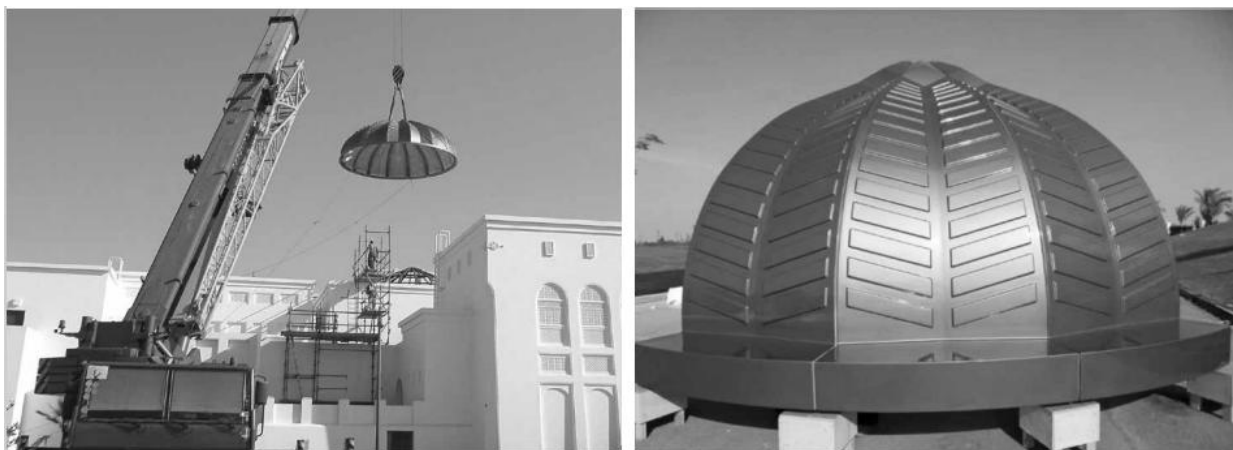
Fig. 5. Convention center 12 m GRP Dome Location: Bahrain Client: Private Engineering Consultants: Gulf House Engineering Main Contractor: NASS Contracting Handover: 2012
