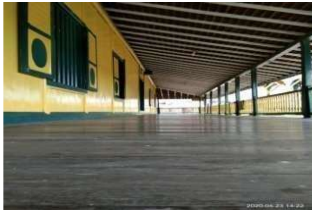
Figure 4. Mosque Terrace Floor
