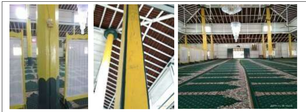
Figure 5. Condition of Main Column and Secondary Column
