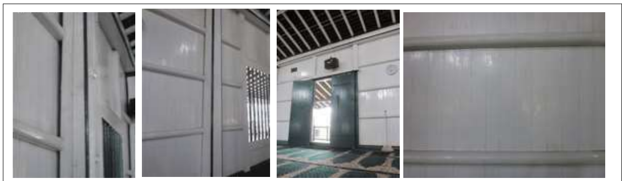
Figure 9. Walls and Wall Beams
