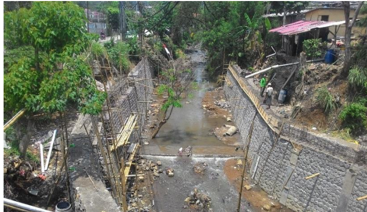
Figure 1. An Illustration of Conventional Retaining Wall Source: Data Survey (2023)
