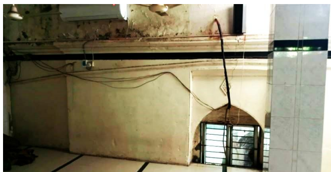
Fig.17 Curved Cornice (Sultani) Converted to Straight Cornice (Mughal), Photographs by 3 rd Author.
