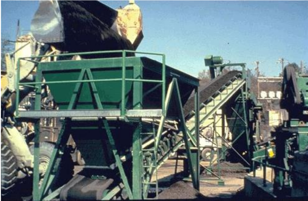
Figure Asphalt batch plant with RAP in feed for hot recycling
