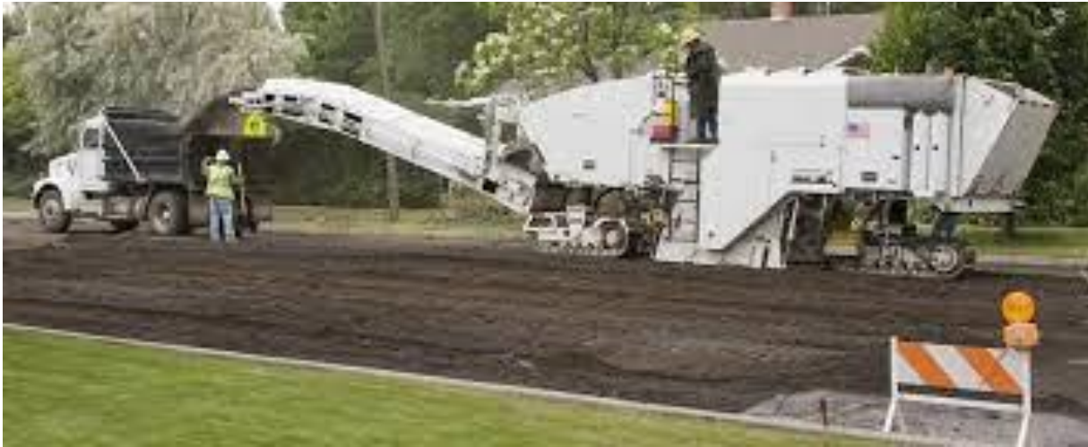
Figure : Pavement rubble from full-depth demolition of roadway
