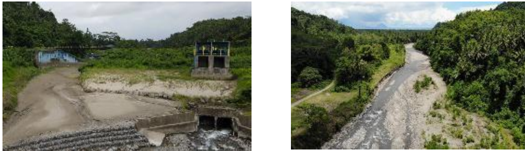
Figure 2. Downstream condition of Oba River and Upstream condition of Sofifi Embung
