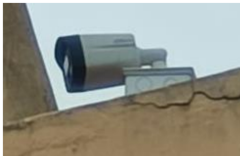
Figure 6: Installed Camera at the Main Gate.
