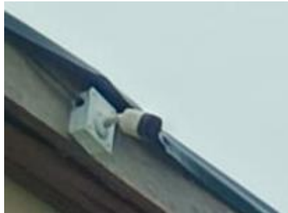
Figure 3: Camera Installed at the Central Administration Building Area.
