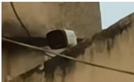
Figure 7: Installed Camera at the Deputy Rector's Office.
