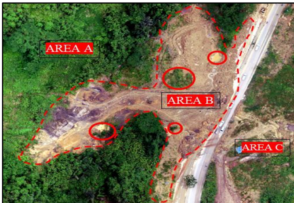
Figure 1. Landslide Zone Division in the Ampera Street Teluk Bajau Area
