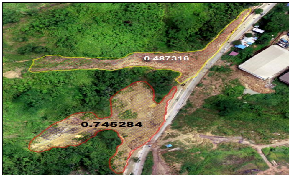
Figure 10. Area of Identified Landslide (Main Landslide and Landslide Affected)
