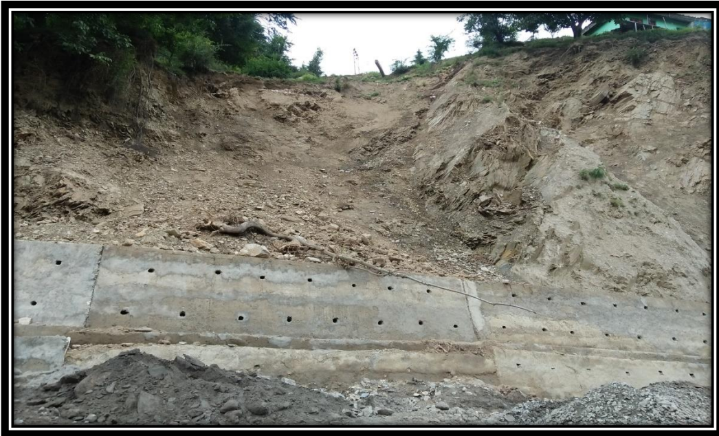
Landslide due to Increase in unit weight of slope material due to increased water content .
