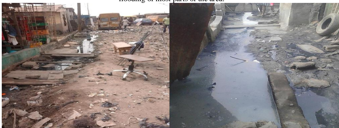
Plate 1: Existing drainage and environmental condition in Makoko
