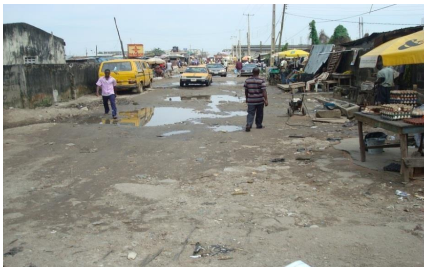
Plate 3: Showing poor road condition with illegal roadside activities Source: Author's Field survey, 2018
