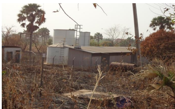
Figure 1. Abandoned Peterson Candy International (PCI) Water Works at Tse-Agberagba (February, 2016).
