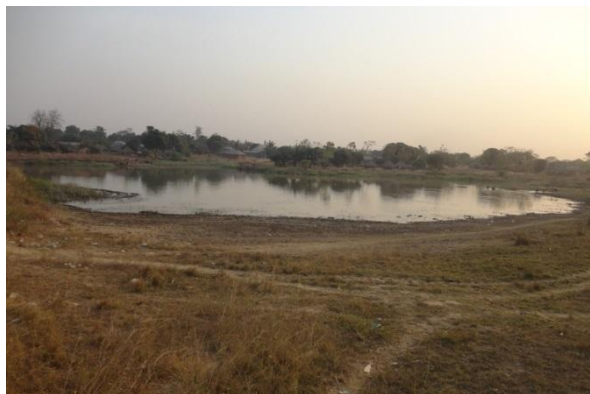
Figure 4. Earth dam at Tse-Agberagba (January, 2017).
