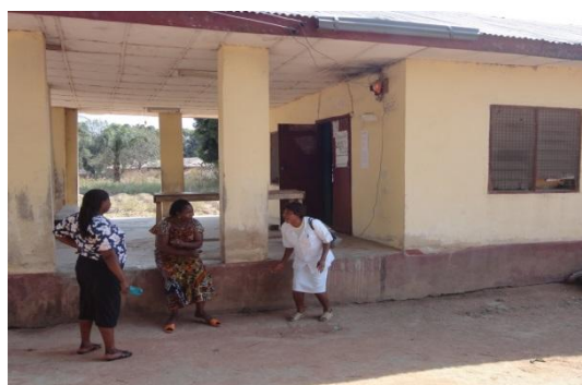
Figure 6. Front view Primary Health Care Centre Korinya(January, 2016).
