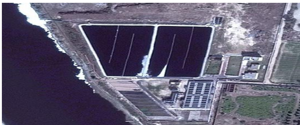
Fig. 9 Sewage treatment plant (STP) Google map
