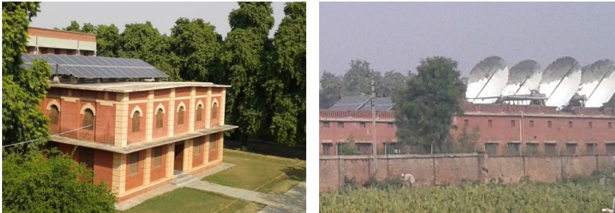
Fig. 5 (a) Solar PV modules for electricity generation (b) Solar power generation and Solar-thermal heating system for hostel cooking.
