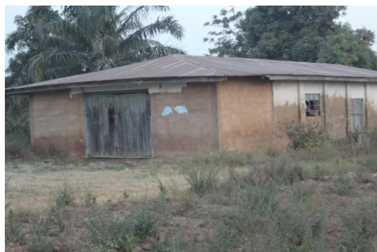
Figure 6. Warehouse at Gungul service centre
