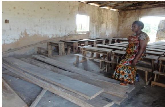
Figure 3. Inside the class room at Korinya service centre
