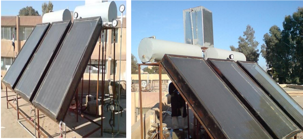
Figure3: The three solar collectors at their installation site
