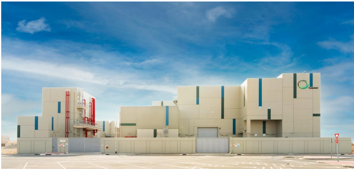
Fig1.1: 132kV Transmission Power Substation
